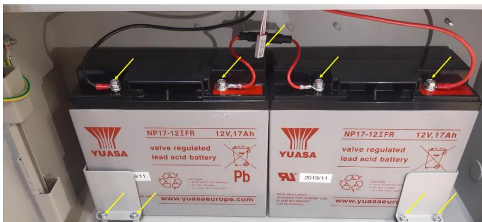
Figure 9: Battery Connection Location for 17 Ah
